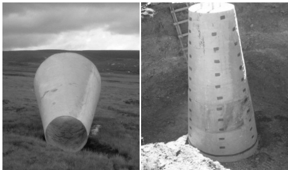
图 1 玻璃钢套筒 图 2 玻璃钢套筒基础 Fig.1Fiberglass sleeve Fig.2 Foundation with fiberglass sleeve
