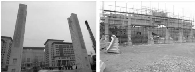
图 7 榫卯构件 Fig. 7 The process of pre-stressed stone archway installation
