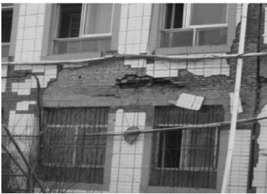
图 16 节点发生破坏 Fig. 16 Damage of the joints
