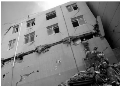
图 17 底层窗间墙破坏 Fig. 17 Damage of the bottom wall between windows
