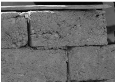
图 21 用泥土堆砌砌块 Fig. 21 Pile masonry with mud
