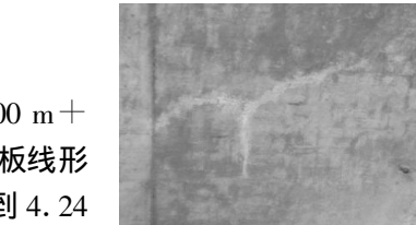
图 1 4 号块腹板裂缝 Fig. 1 Cracks in the webs of block 4
