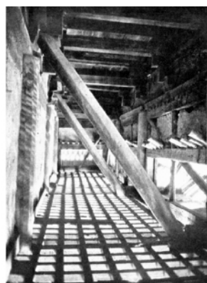
(a) Transverse diagonal bracings
