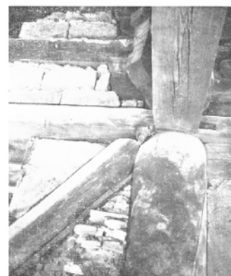
(b) Longitudinal diagonal bracings
