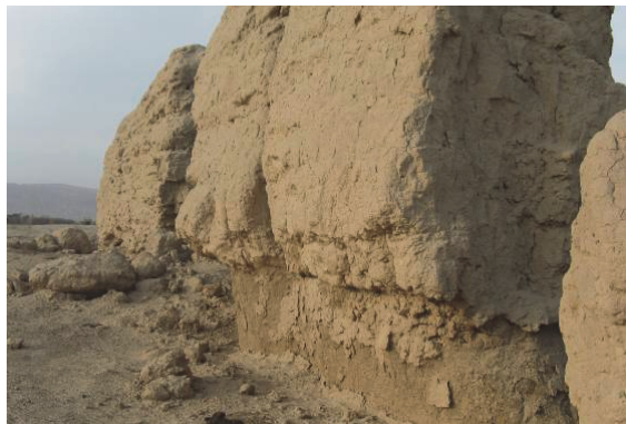
图1 墙体根部掏蚀凹进 Fig.1 Wind erosion of wall root
