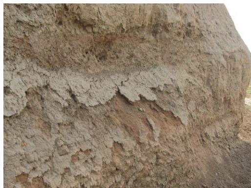
图2 墙面风化剥落 Fig.2 Wind erosion of wall surface
