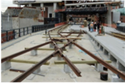
图 3 保留铁轨施工 Fig.3 Construction of the reserved railway
