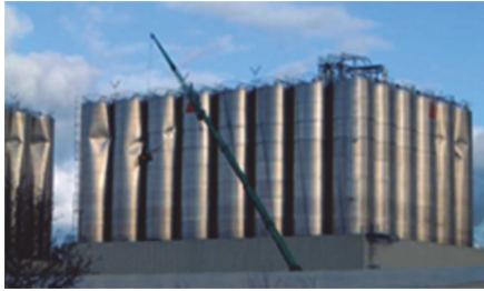
图1 薄壁圆柱壳体在在外部压力作用下的屈曲破坏 Fig.1 Buckling phenomenon of thin cylinders under external pressure
